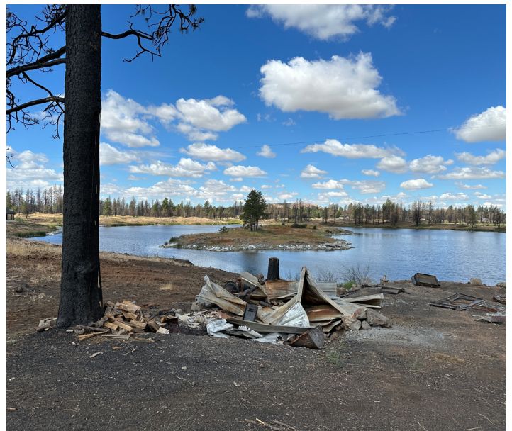
Structure loss after the 2023 Gray Fire, WA (photo: Cat Edgley)
