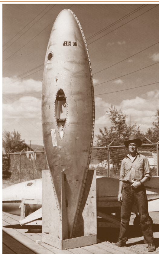
▲ A 310-gallon tank bomb retrofitted with plywood fins to assist with delivery, Missoula, MT, 1946. Forest Service photo.
