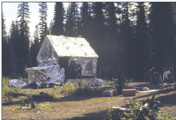
Figure 9S-5f —Crews commonly wrap back country structures with fire shelter cloth to minimize structure ignition.
