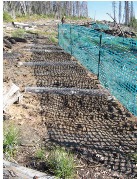
Figure 5. Ulm Peak installation (September, 2009) using snow fence for shade.
